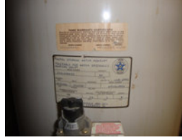
#2655 Older water Heater
