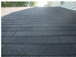
#2669 View Of Roof
