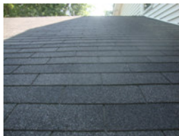
#2669 View Of Roof
